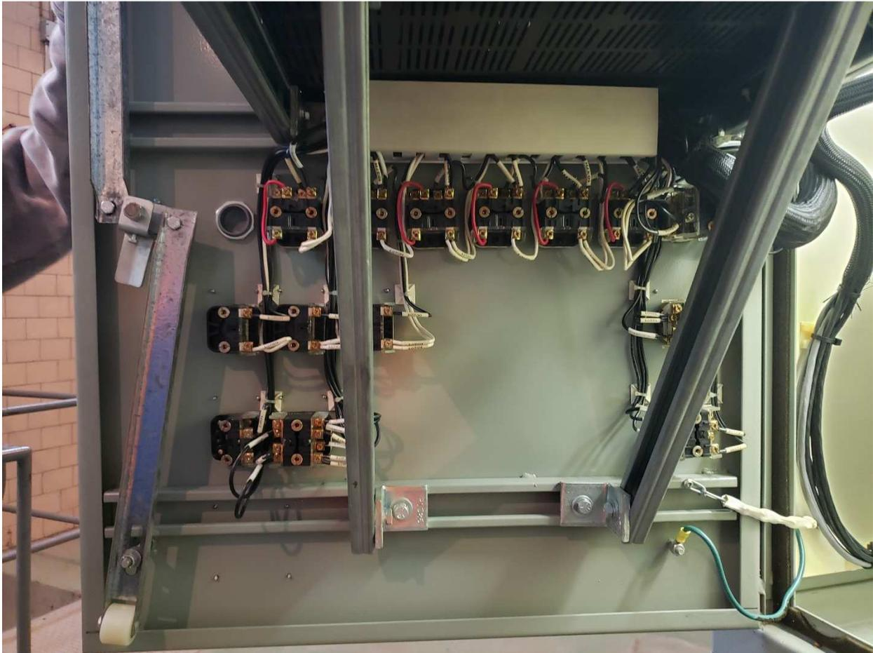
PHOTOGRAPH 3: Tache Booster Pumping Station – Pump PP-1 Local Control Panel LCP-1 – Bottom Interior Door View.
