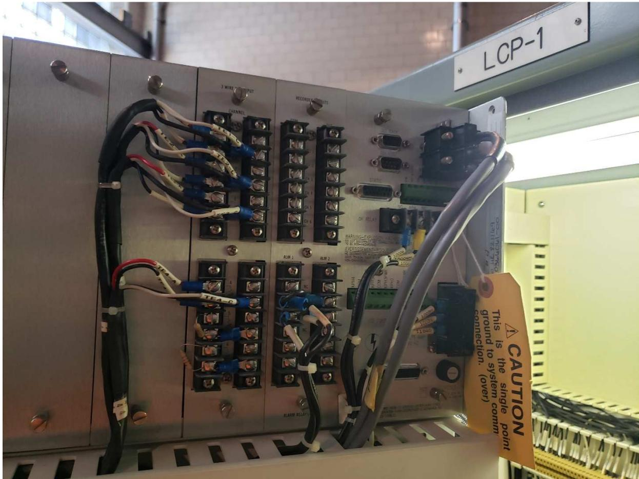
PHOTOGRAPH 2: Tache Booster Pumping Station – Pump PP-1 Local Control Panel LCP-1 – Top Interior Door View.
