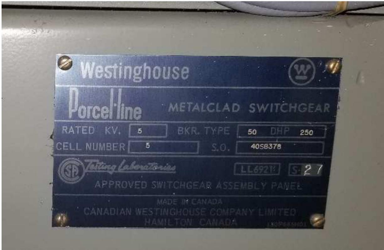
PHOTOGRAPH 5: McPhillips Regional Pumping Station – Main 4160V Switchgear SGR-M1 nameplate
