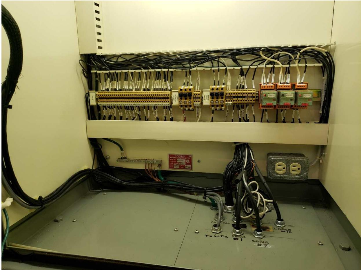
PHOTOGRAPH 4: Tache Booster Pumping Station – Pump PP-1 Local Control Panel LCP-1 – Inside View
