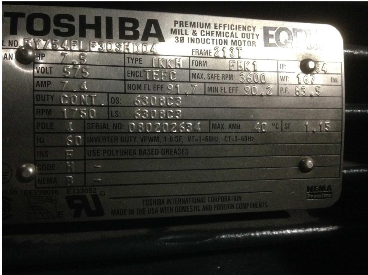
PHOTOGRAPH 8: McPhillips Regional Pumping Station – Air Compressor AC2 Motor Nameplate
