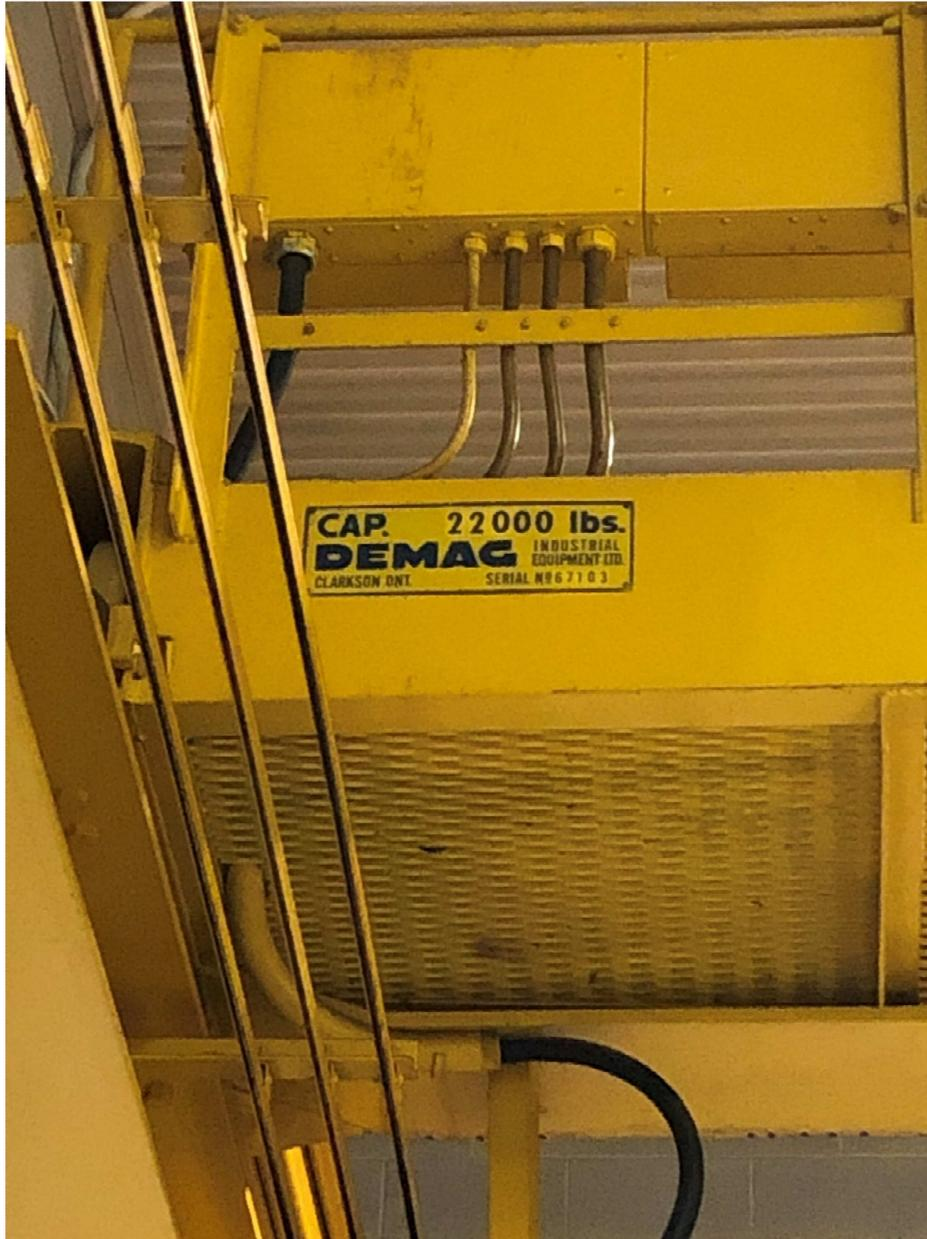
PHOTOGRAPH 11: McPhillips Regional Pumping Station – Crane Nameplate Information
