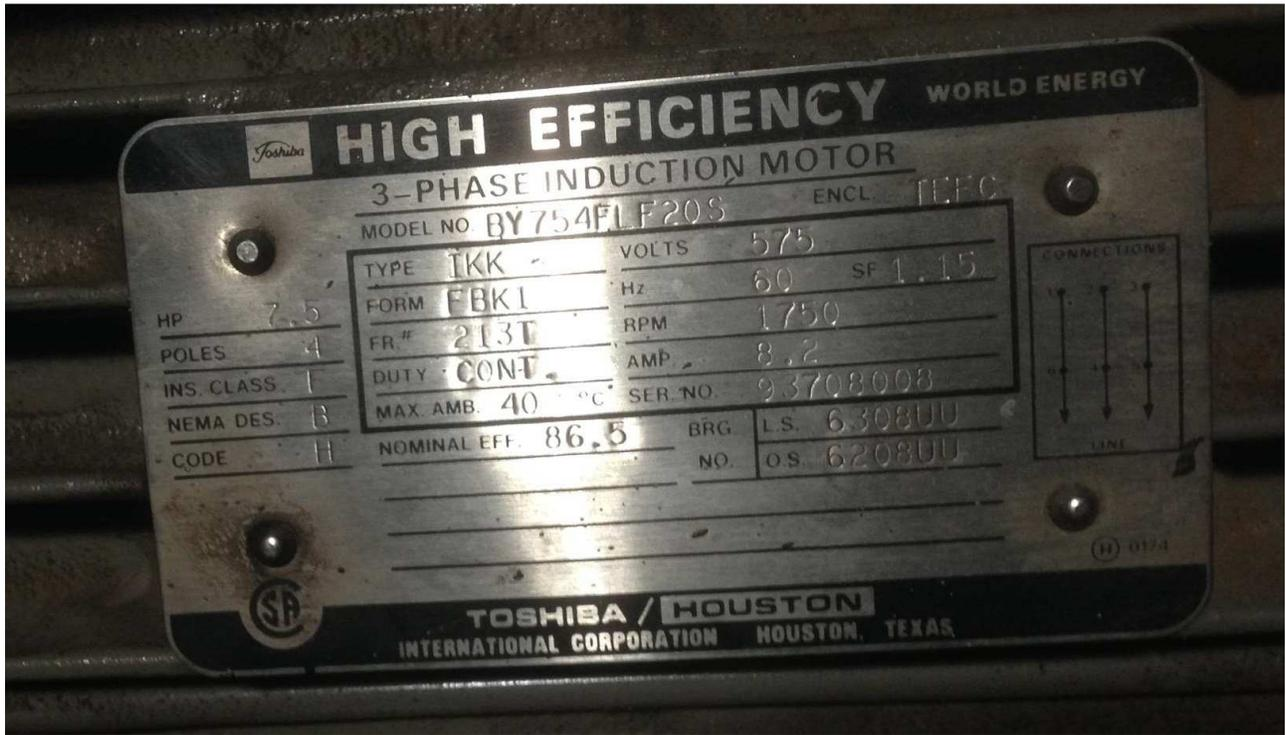
PHOTOGRAPH 6: McPhillips Regional Pumping Station – Air Compressor AC1 Motor Nameplate
